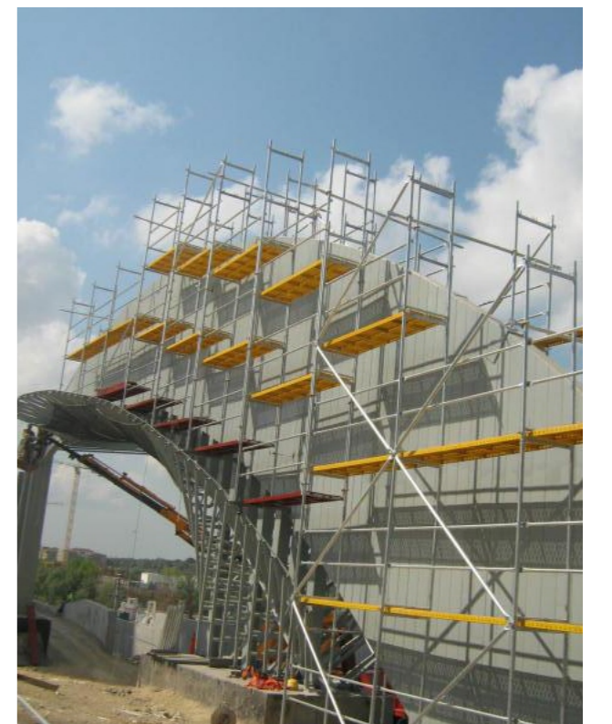
ERBA İNŞAAT - BOSPHOURS CITY
