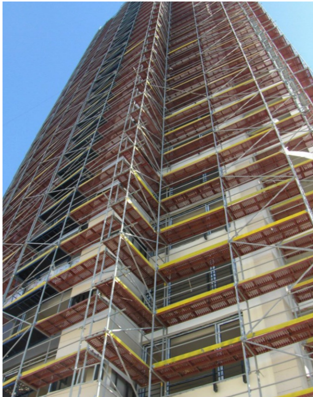
ERBA İNŞAAT BOSPHOURS CITY
